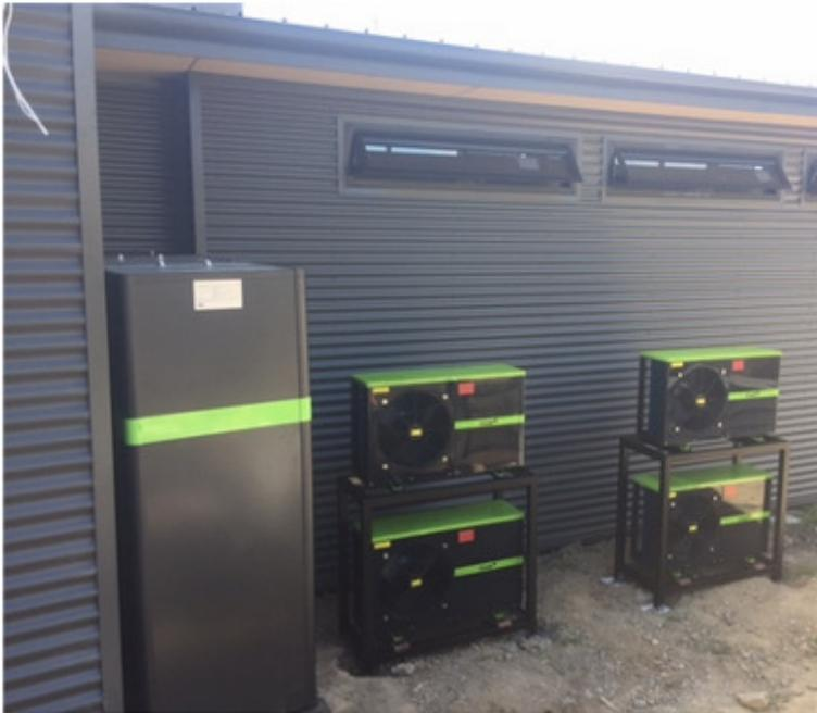
Pictured above the Tivok 30.4kW Heat Pump system in the process of installation by Mark McCormack one of our preferred installers. Note the steel mounting brackets keep the Heat Pumps independent of any wall , for a full Tivok Product Profile [PDF: download](#)
